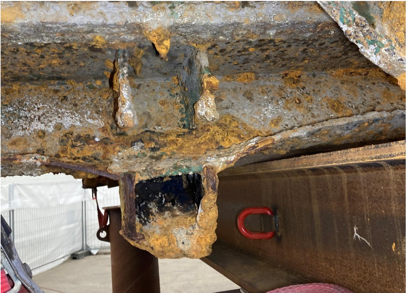
Figure 4. Port side lower ramp side lock box.
