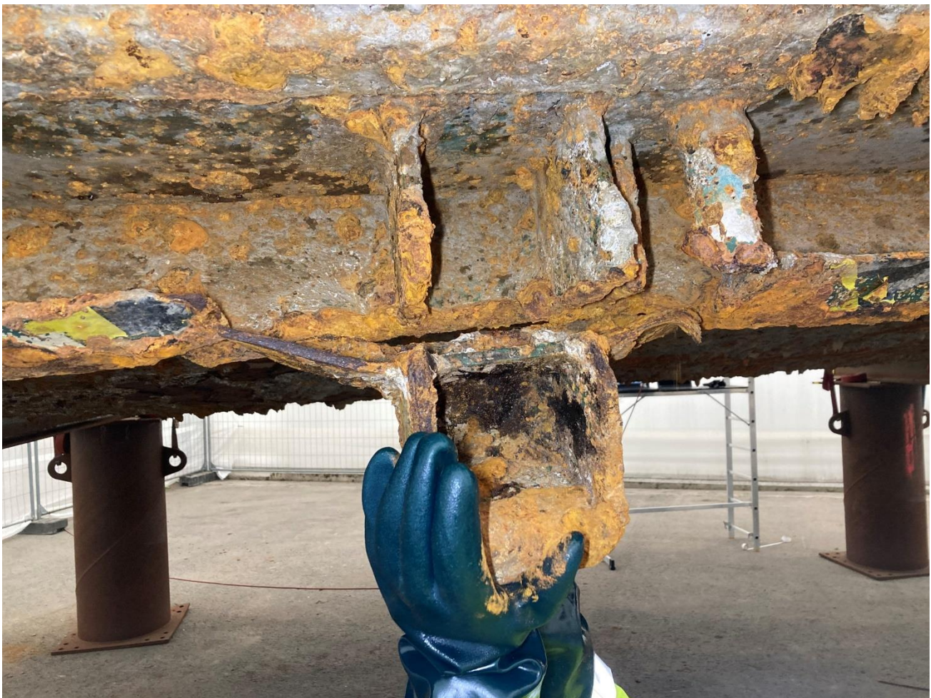
Figure 3. Port side upper ramp side lock box.
