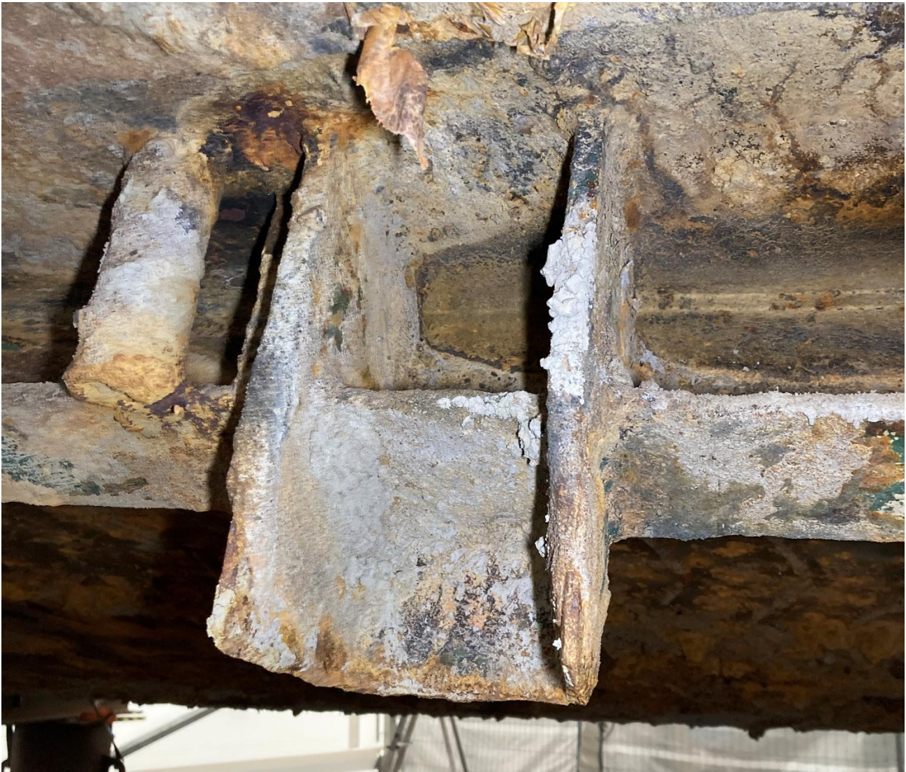
Figure 5. Starboard side upper ramp side lock box.
