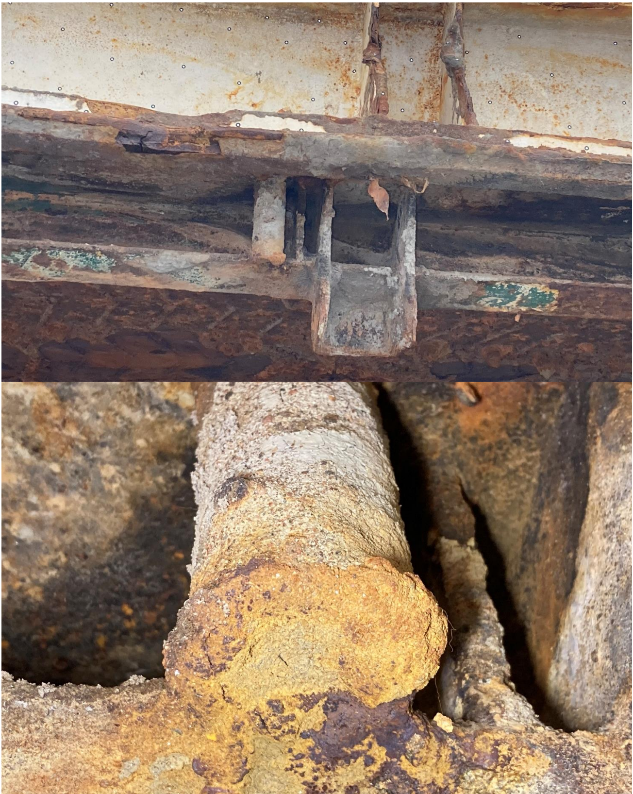
Figure 10. Starboard attaching position for railing (2 in Figure 8).
